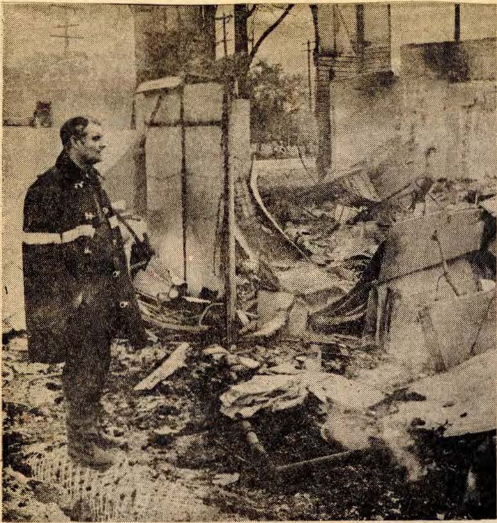
FIRE SCENE — Port Stanley Fire Chief John Vary inspects the ruins of the Bath House and Cafeteria early this morning after flames swept through the tinder-dry, historic structure. One firefighter was injured in the blaze.
